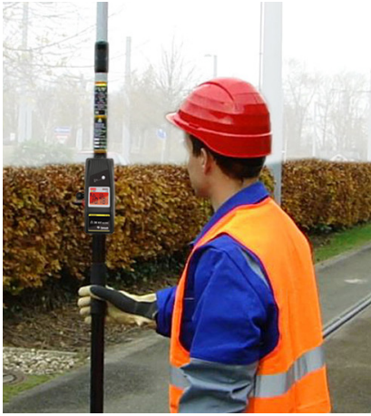
Test at overhead line
