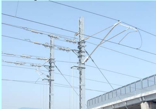
Railway Electrification: 15 – 25 kV c.a.
